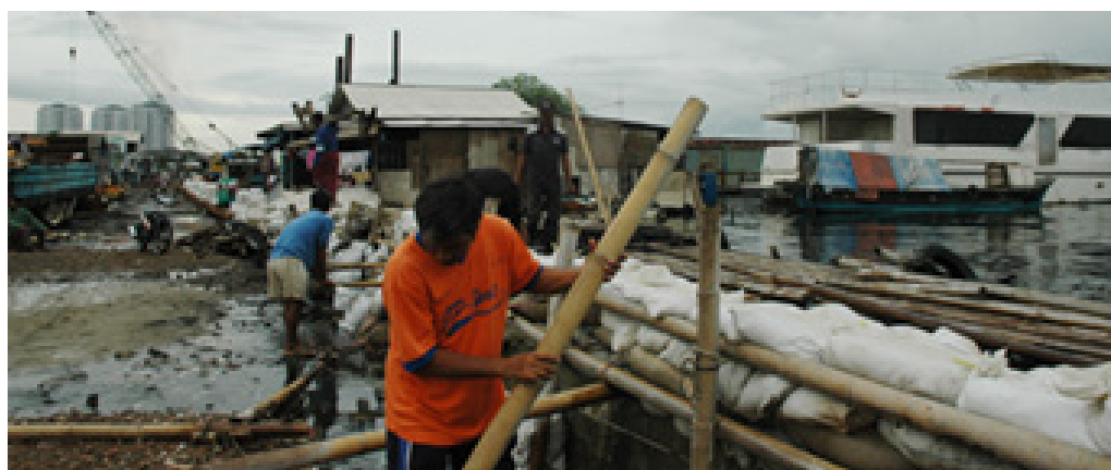
Jakarta dike reinforcement with sandbags and bamboo during the 2009 flood.
