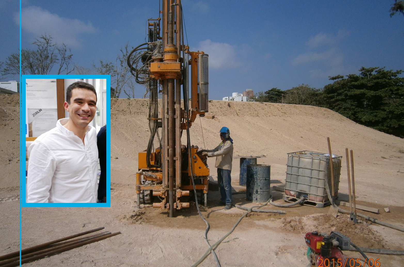
SPT Operation Plus Boreholes - 20 story building, Barranquilla
