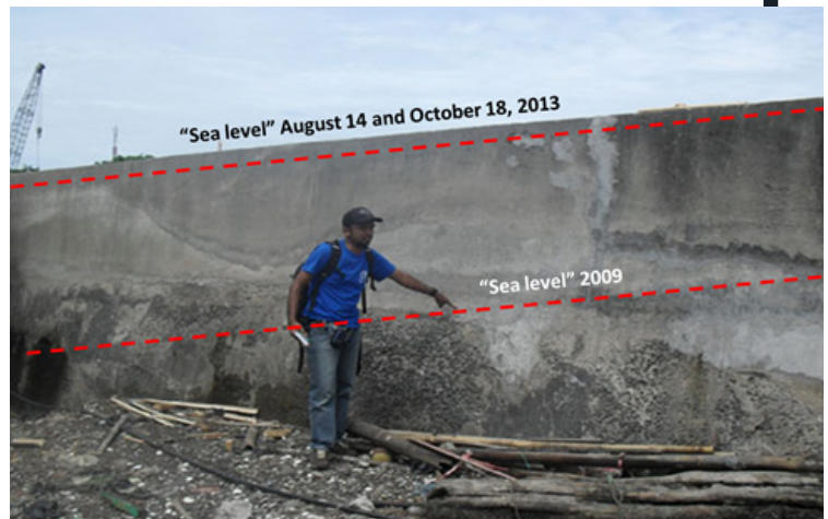
Dike at Pluit, at the coast of Jakarta. People are living more than 2 m below the sea level. This wall has been raised in 2016 after a flood and flooded again in 2017.
